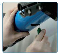
• Remove debris and deburr cut edges.
