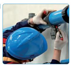
• Mark the pipe where the hole for the quick drop connector will be installed.
